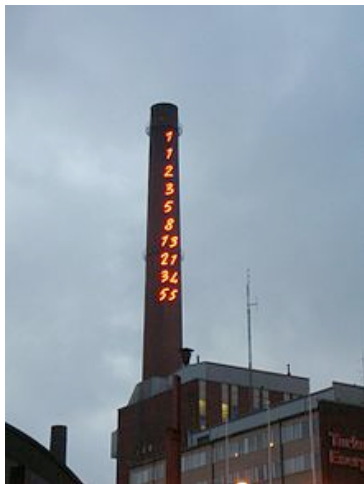
Figure : The chimney of Turku Energia in Turku, Finland, featuring the Fibonacci sequence in 2m high neon lights (Mario Merz, 1994).
